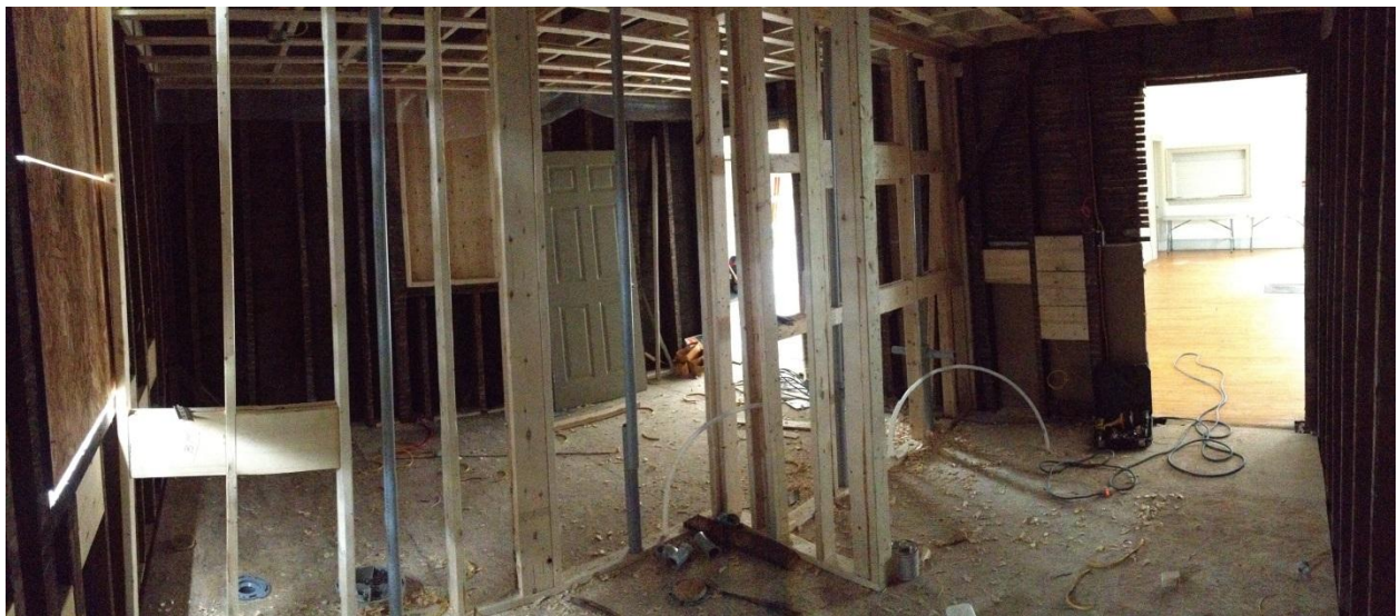
(Hall bathrooms: Sealed window openings, Framing and Plumbing)
