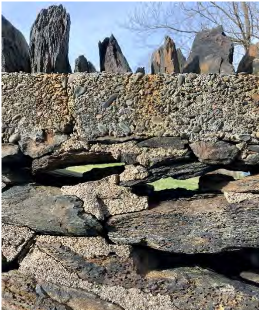
Left: The Gerrish Street wall prior to restoration. Note the missing stones and mortar from previous attempts at repair.
