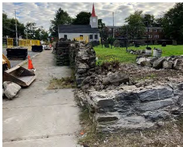
Left (foreground): the deconstructed 1950's extension to the Gerrish Street Wall. Until the early 20 th century, a house stood on that spot. It is thought that the wall extension (added in the mid-20 th century) was built on top of the foundation, hence the setback between the two wall sections.
