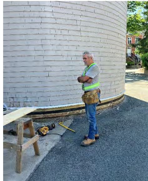
The skirting boards around the chancel are replaced
