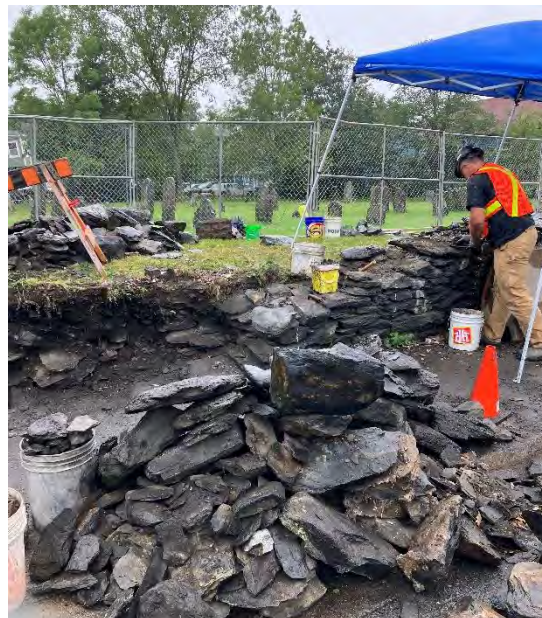
Left: The Gerrish Street wall prior to restoration. Note the missing stones and mortar from previous attempts at repair.
