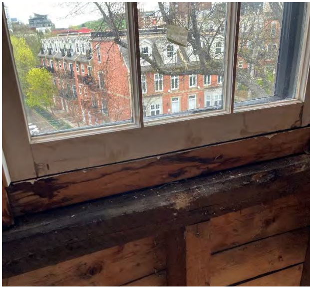
A south-side clerestory window with drywall removed
