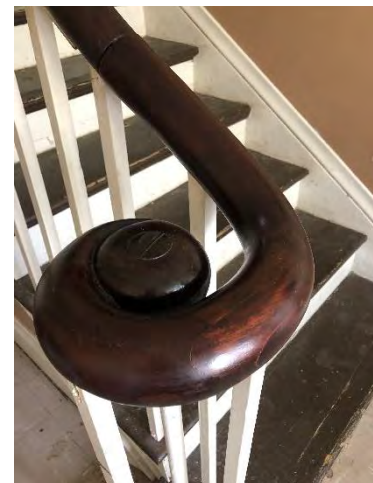
The repaired bannister
