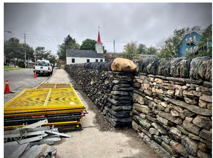
Left (foreground): the deconstructed 1950's extension to the Gerrish Street Wall. Until the early 20 th century, a house stood on that spot. It is thought that the wall extension (added in the mid-20 th century) was built on top of the foundation, hence the setback between the two wall sections.
