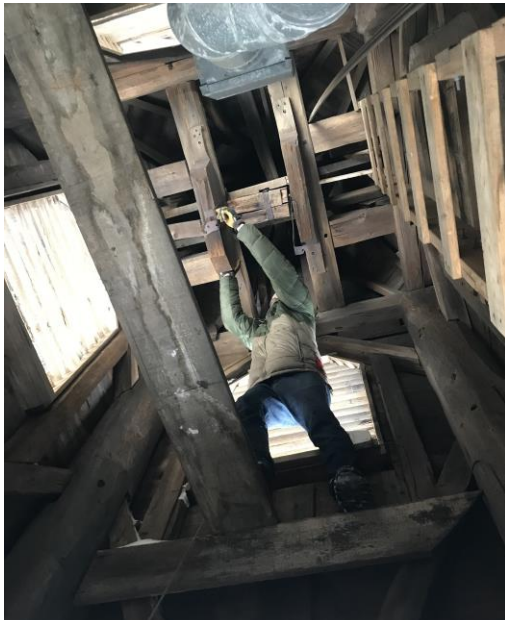
Evan prepares to remount the LDC bell in the steeple
