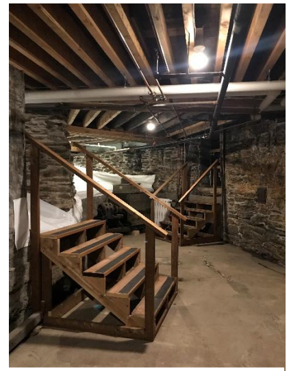
Access stairs, constructed for ease of maintenance.
