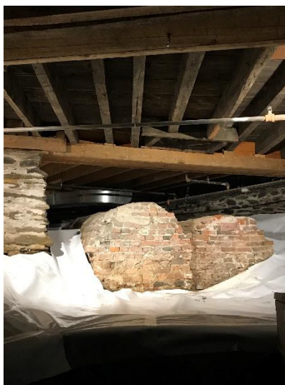
The graves of Col. JFW des Barres and his wife, Martha Williams, illuminated by new display lighting, and showing the newly-installed vapour barrier (white)
