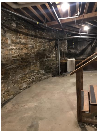
The cleaned-out church basement
