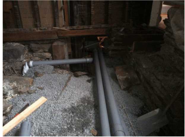
(Conduit and drains looking East)
