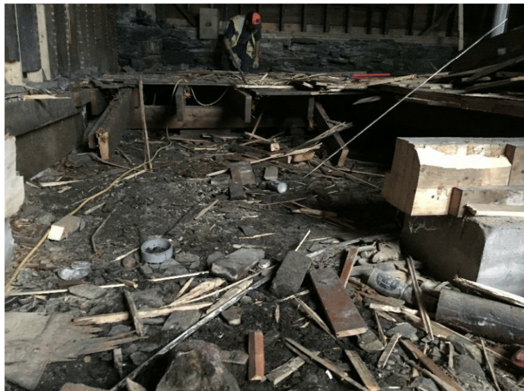
(Demolition of the West side of the music room floor)
