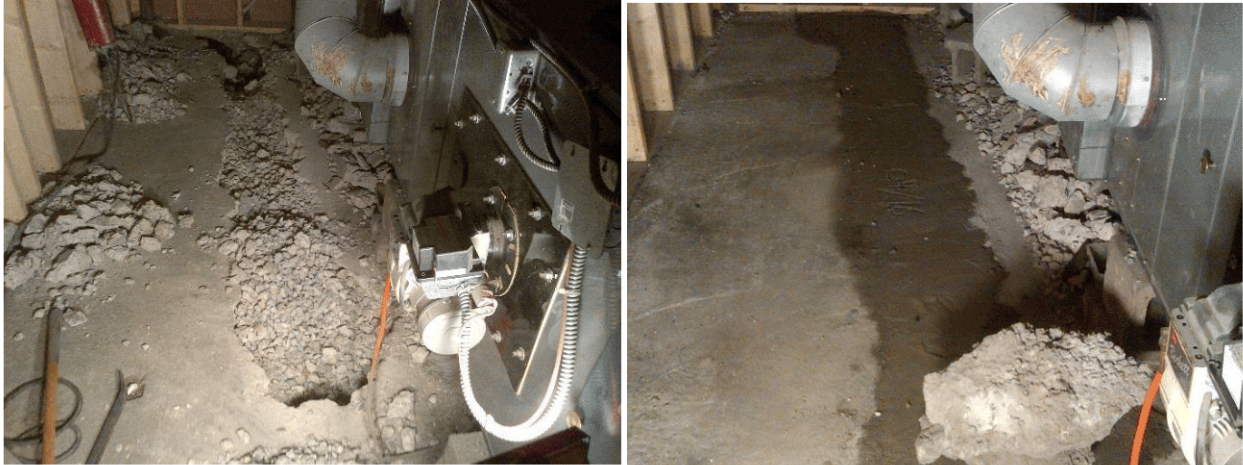
(Demolition and installation of floor drain in boiler room)
