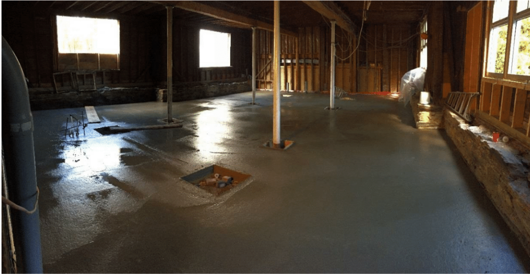
(Freshly poured slab)
