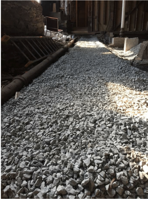
(Gravel Bridge for conduit looking West)
