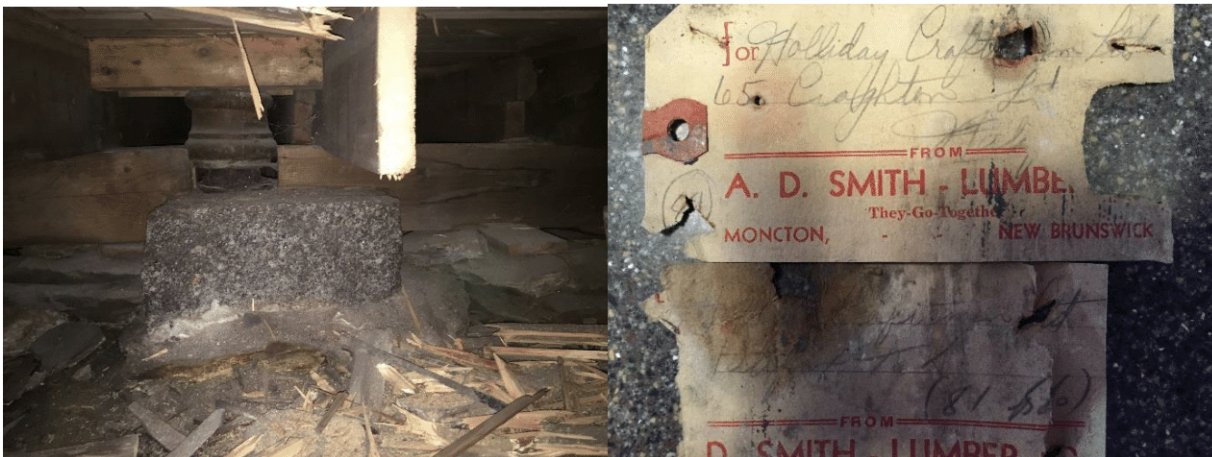
(Left: Granite Slab and base of iron posts, Right: Lumber Delivery Artifacts)
