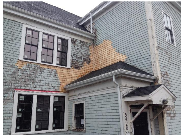
Water infiltration repair
