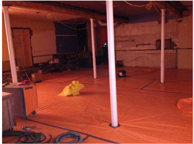
Asbestos Abatement in the Music Room
