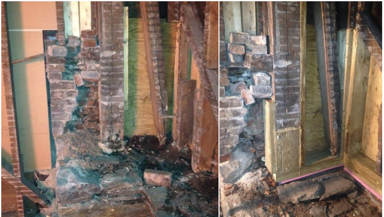
Left: Supporting post showing its age, Right: Supporting post after repair
